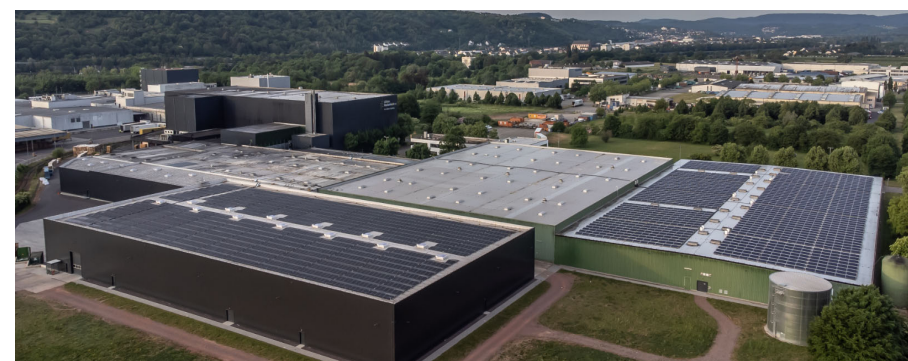
Photovoltaic system in Trier
